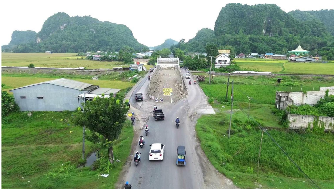
Figure 2. Construction of the Sapanang Overpass
