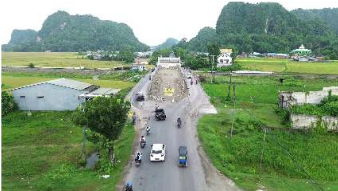
Figure 2. Construction of the Sapanang Overpass
